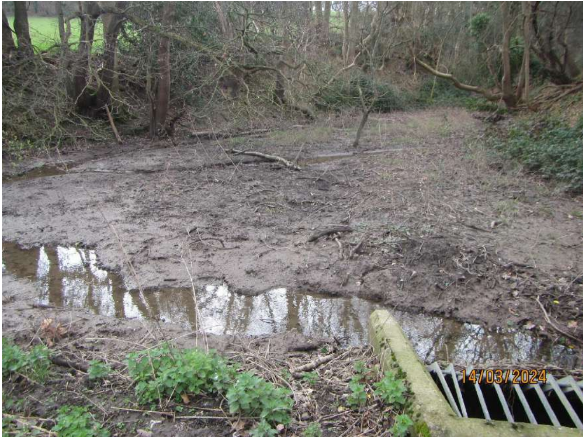
Photograph 13. Culvert from the woodland to the ditch
