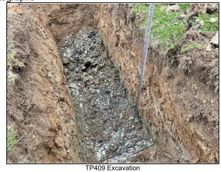
Remarks: Unable to advance the hole further than 1.20m. No groundwater encountered. On completion trial pit was
