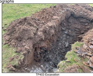
Remarks: Unable to advance the hole further than 1.55m. No groundwater encountered. On completion trial pit was backfilled with arisings.
