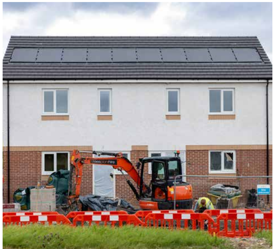
Work is almost complete at New Inn, Sandycroft
